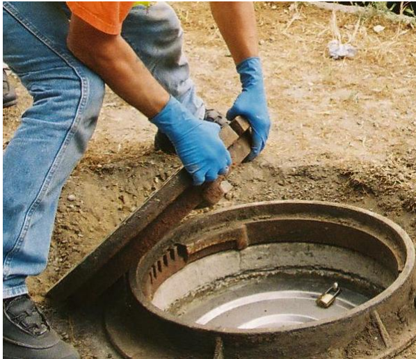
1) REMOVE CAST IRON COVER.
