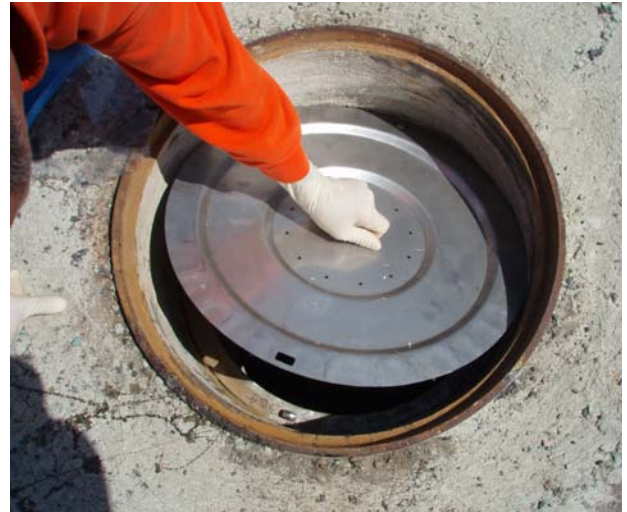
2) REMOVE PADLOCKS, TURN EYEBOLTS TO ALIGN WITH SLOTS IN INNER COVER, AND LIFT OUT THE INNER COVER.
